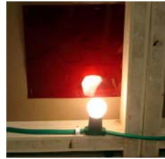
Floor light construction
