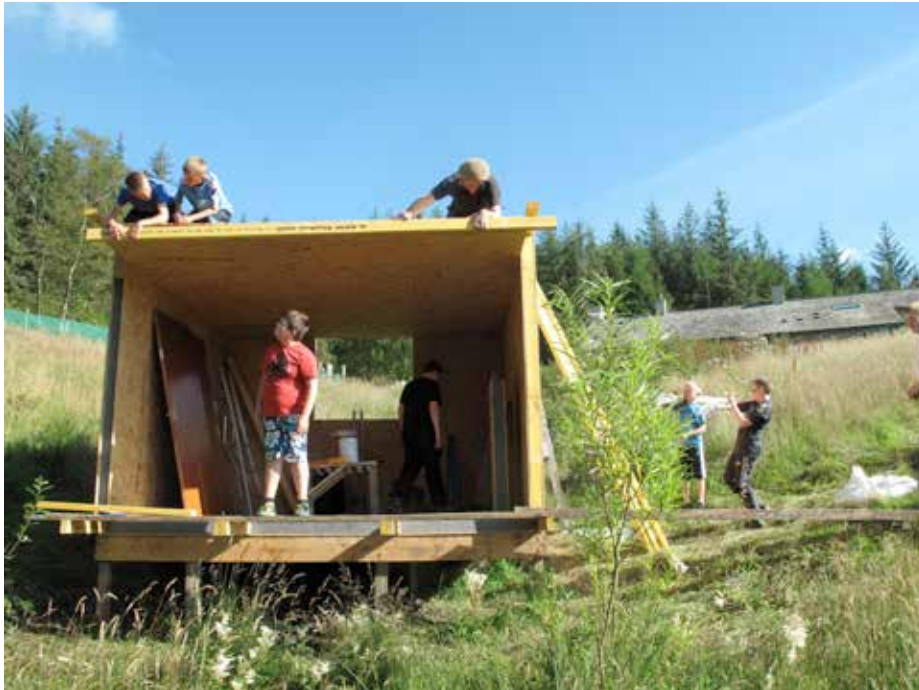
Building the shed. Courtesy of Grizedale Arts
