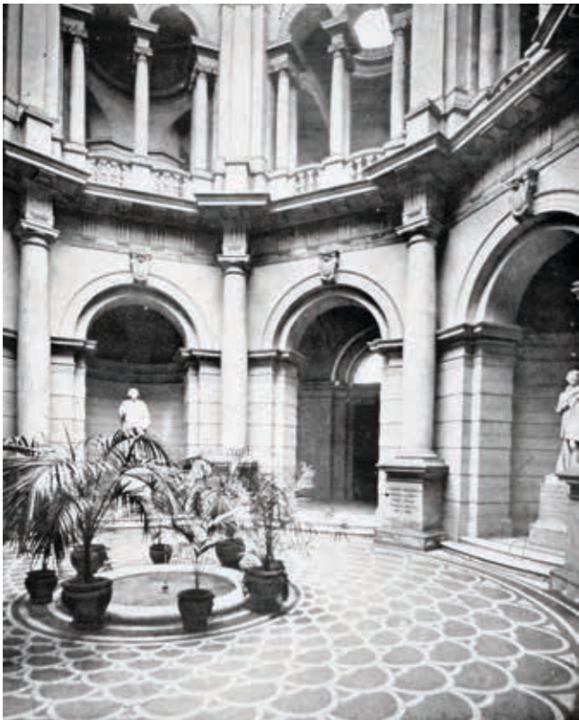
The Rotunda with the original floor and fountain before it was demolished
